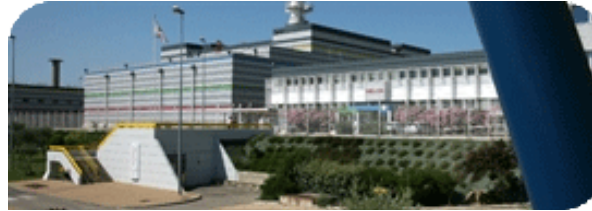
MELOX - MOX fuel fabrication plant
